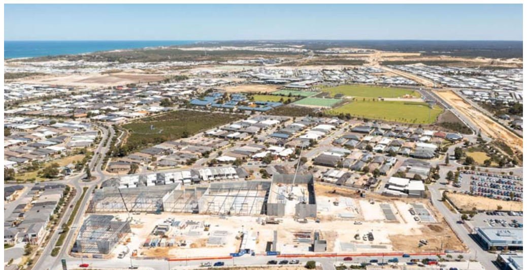
Construction progress November 2021
